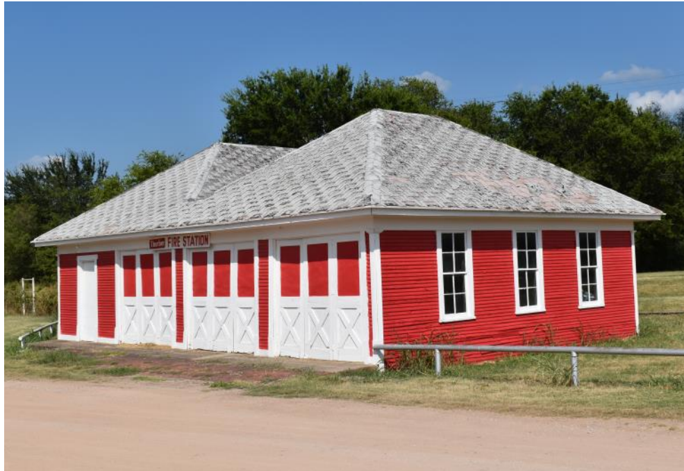
Another original building is this fire station very close to the smokestack and across from the restaurant.
