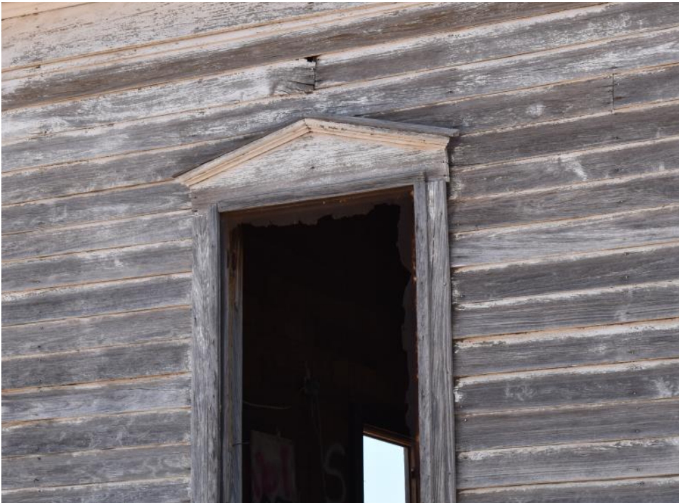
Detail of window from the east side of the building.
