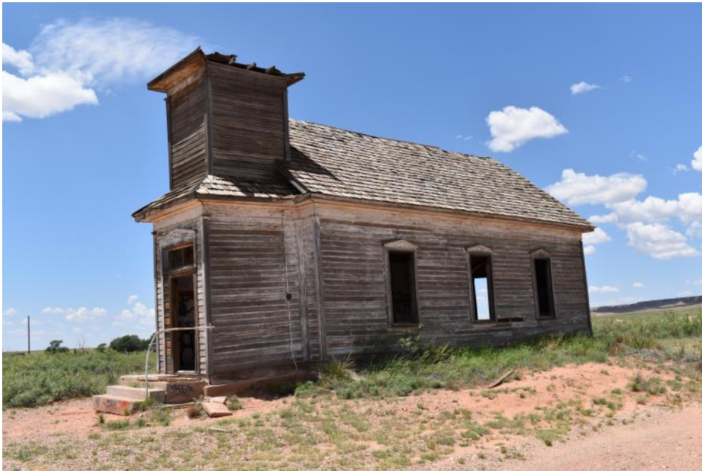
View from the southeast.
