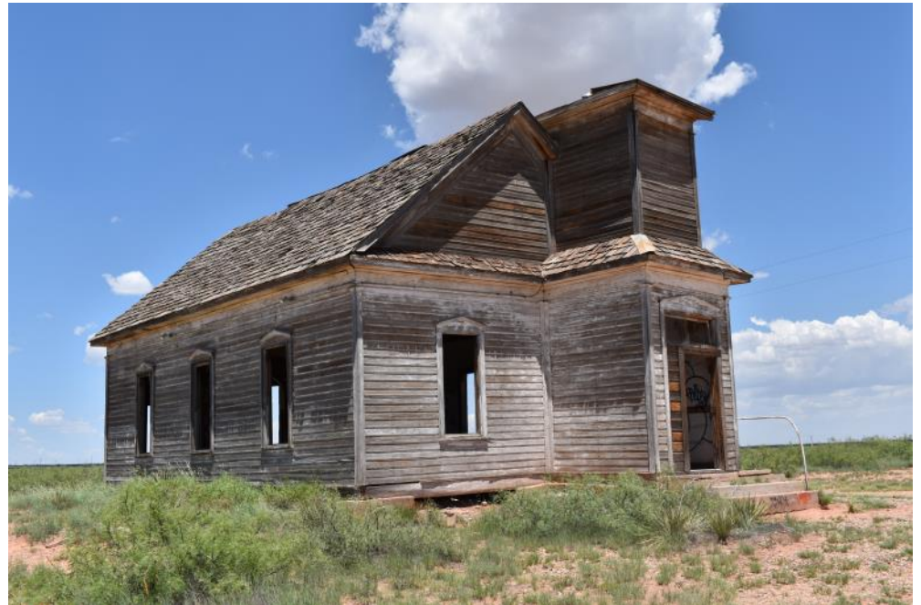
View from the southwest.
