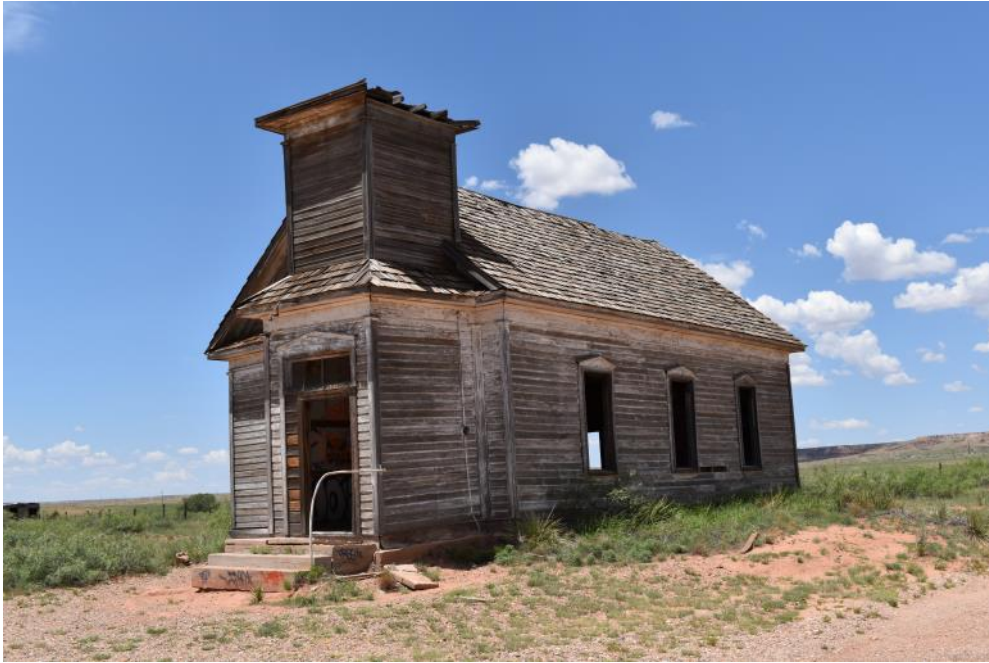
View from the southeast.
