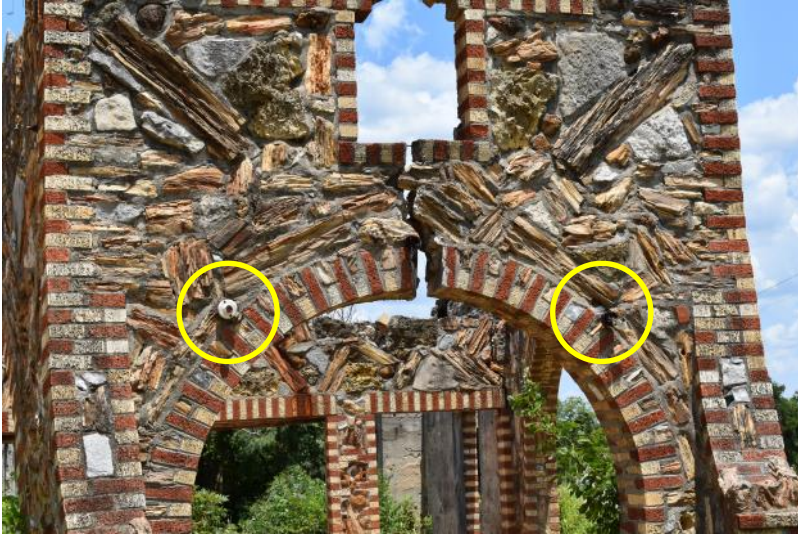
The building looks like it was built first, then electricity added later, in a knob and tube style. The front (above) shows two lights, while each side of the large arch has six lights each. The two pronged outlet looks like it was added.
