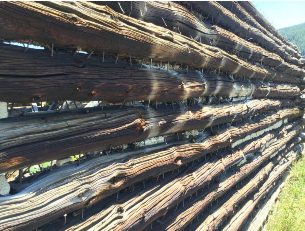
Another view of the logs showing the nails that held the chinking.
