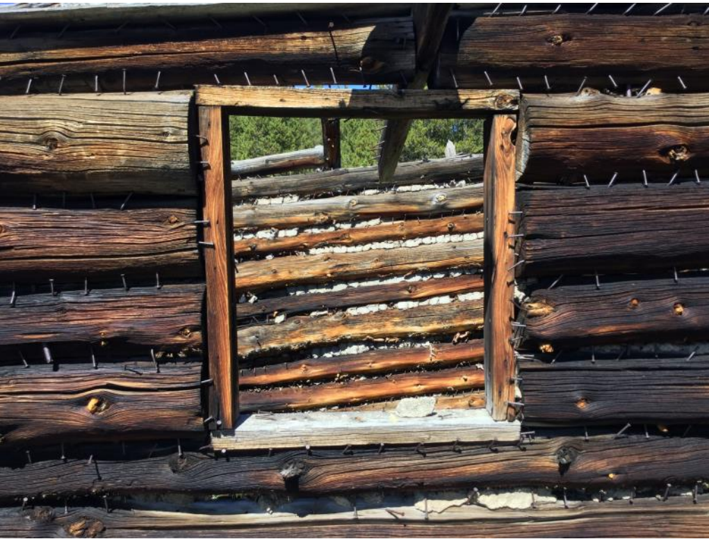
The windows in this cabin are firmly held by boards that become an integral part of the structure.
