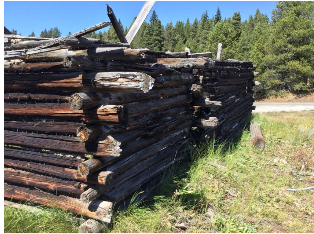
Like with many log cabins, the corners show a good overlap.
