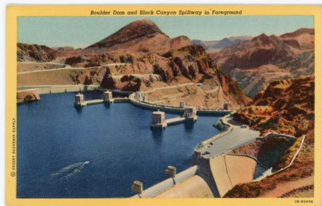
Boulder Dam and Black Canyon Spillway in Foreground
