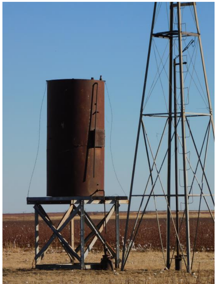
Unusual fabricated steel tank.
