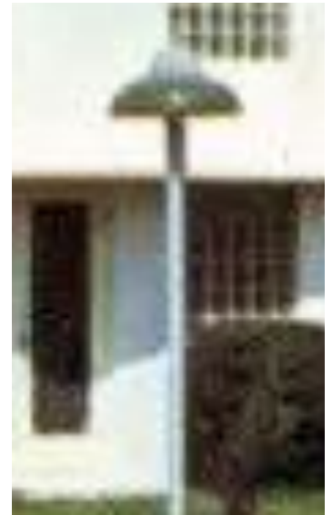
These light poles with a characteristic green cover were in several places in the front.
