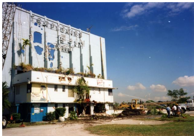
The dozer made much more efficient progress.
