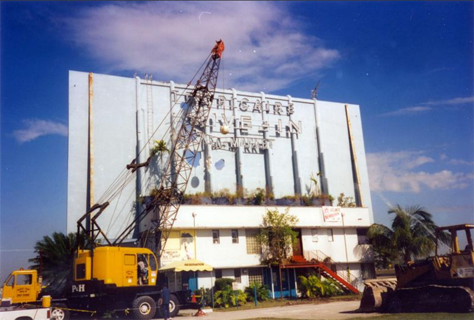
The wrecking ball was not very effective in that it mostly bounced off the wall and just made Swiss cheese of the wall!
