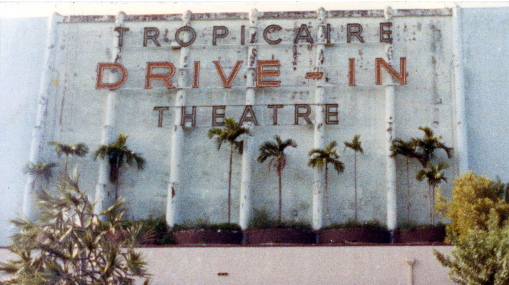
The original neon sign within channel lettering on the front of the screen. The hanging garden was below originally containing palm trees and other tropical plants. Many of the palm trees were still there in the 1980s. Photo by: Robert-George de Stolfe
