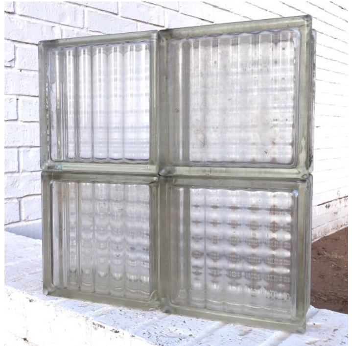
Original glass blocks from the Tropicaire Drive-In Theatre, originally installed in 1948-1949.
