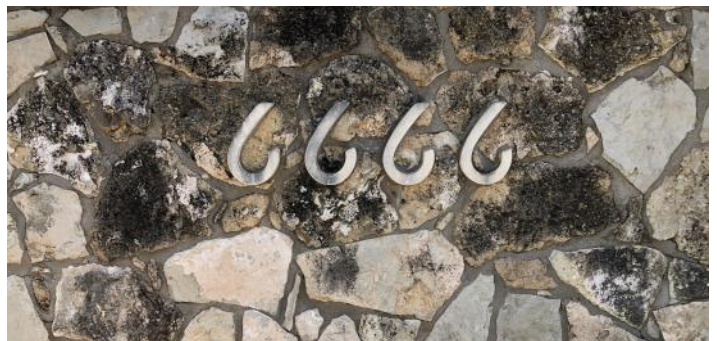
The 6666 brand on the rock wall of the entrance.
