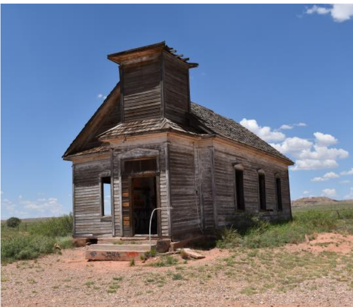
The old Presbyterian church in Taiban, New Mexico
