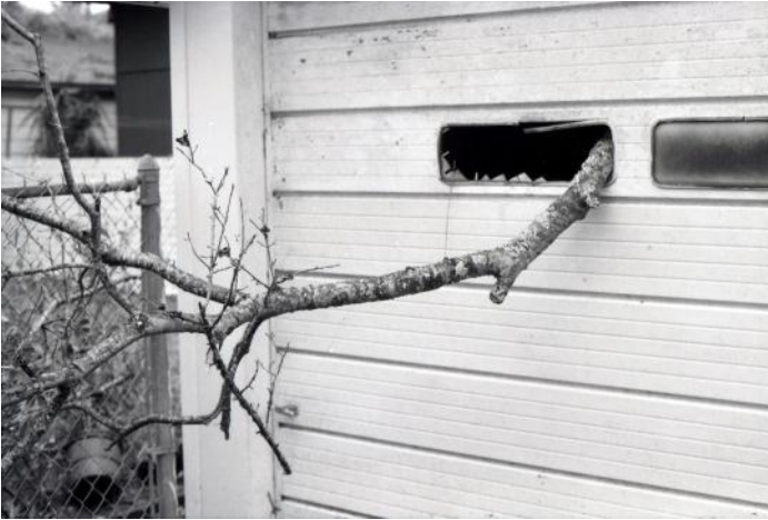
The only damage to the garage was this window.
