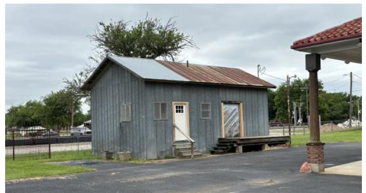
Another structure behind depot near the railroad tracks.
