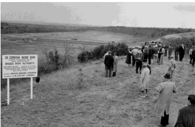
Site of the future dam in 1966 that would create Lake Granbury. (Brazos River Authority)
