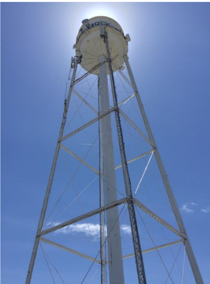
Shamrock water tower, 176' high, completed in 1916, 75,000 gallons.
