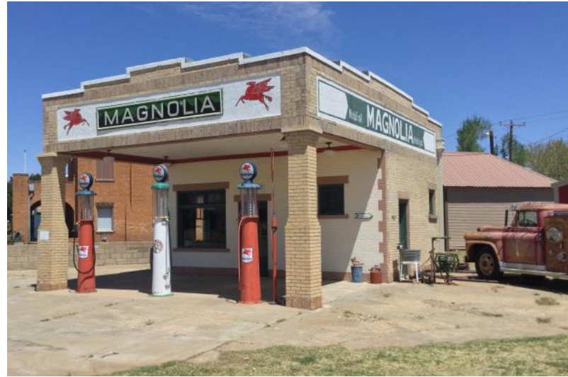
Restored Magnolia Gas Station in Shamrock, Texas
