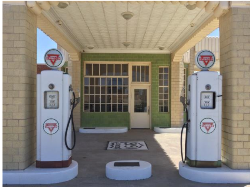
One gas bay of the Tower Station.
