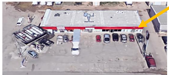
This strange 3D rendering from Google Earth shows the Rudd's building with a gas station, feed store, and an empty space where we had Bible studies. The building was recently torn down for road expansion.
