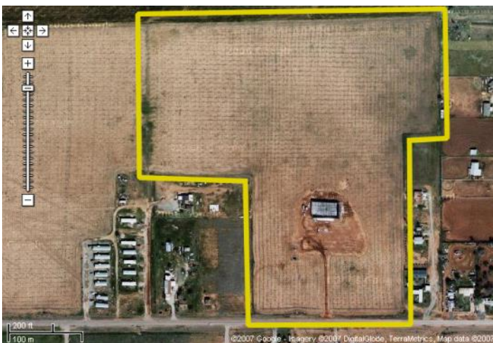
The new church land was in NW Lubbock, outlined in yellow. It was an old cotton field. Here, you can see the steel trusses in place.
