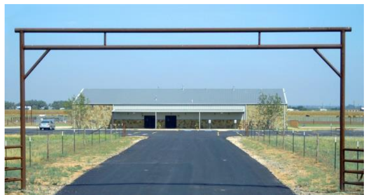
Construction of the new church building started in January and completed in time for the Fourth of July in 2005. A little later, a pipe entrance framed the front of the property.
