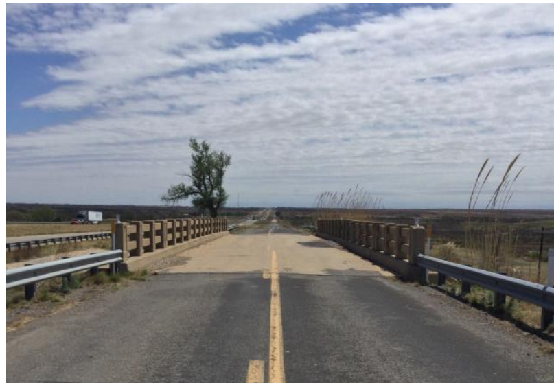
Route 66 bridge about 8 miles east of Shamrock.
