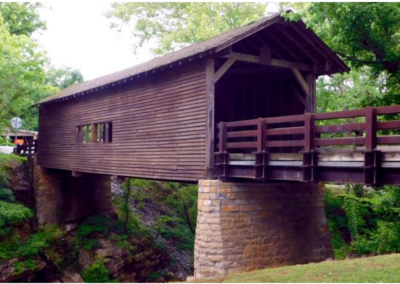
Harrisburg Covered Bridge. 5.24.22.
