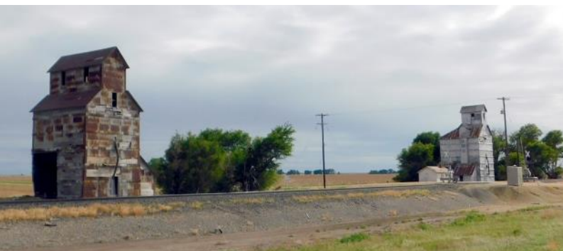
Found these two square silos out on the plains of southern Kansas. 6.1.22.
