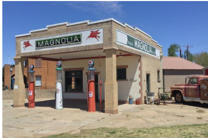
Restored Magnolia Gas Station in Shamrock, Texas
