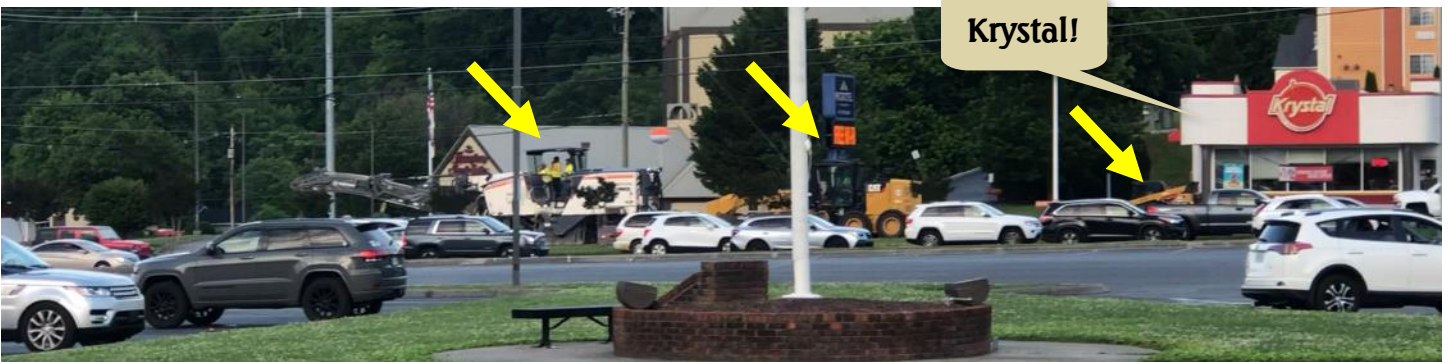
Convoy of road pavers
