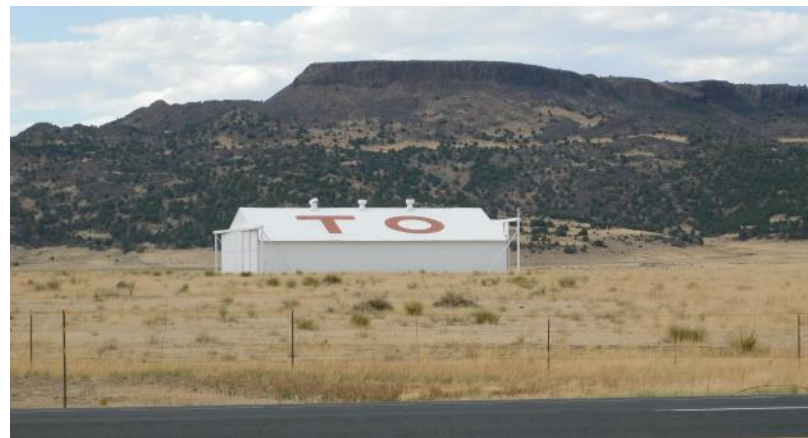
Hangar on the T.O. Ranch.
