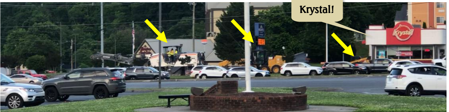
Convoy of road pavers
