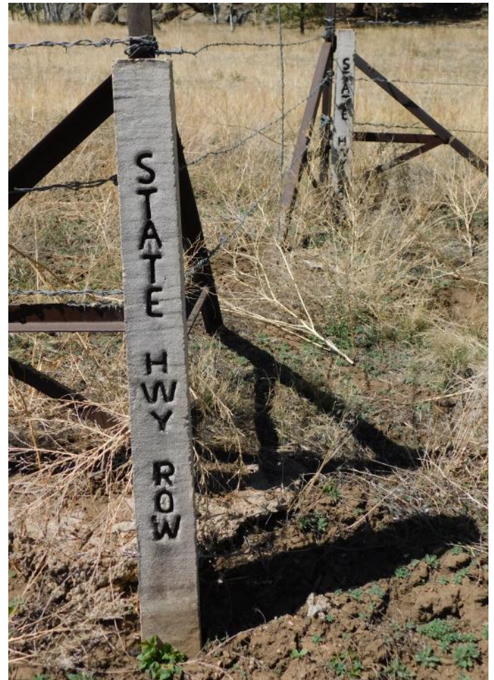
Old concrete highway markers.
