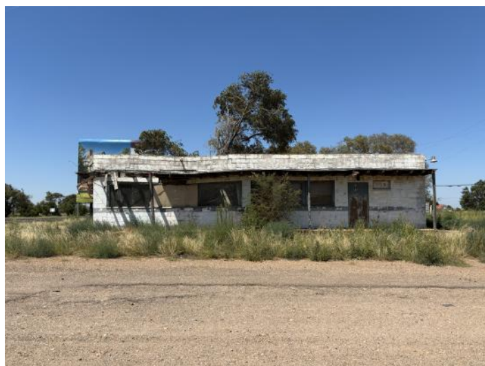
Side of building as of Wednesday, August 6, 2025.
