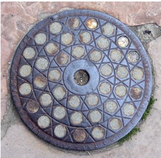
Old manhole covers are very interesting! Here are two in Leadville. There are several like the one to the left around town. The little circles originally had glass to let in light to the underground. Both have the name of the manufacturer around the edge.
