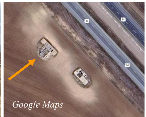
Overhead photo of structure from Google Maps.
