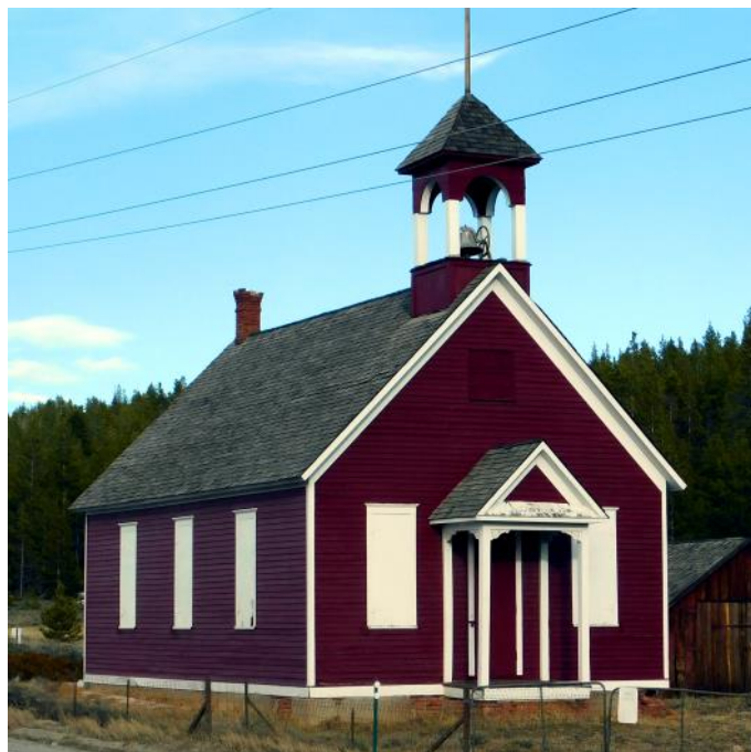
This is a schoolhouse. Located a few miles west of Leadville, the Malta school was built in 1902 and was in continual use to 1945.
