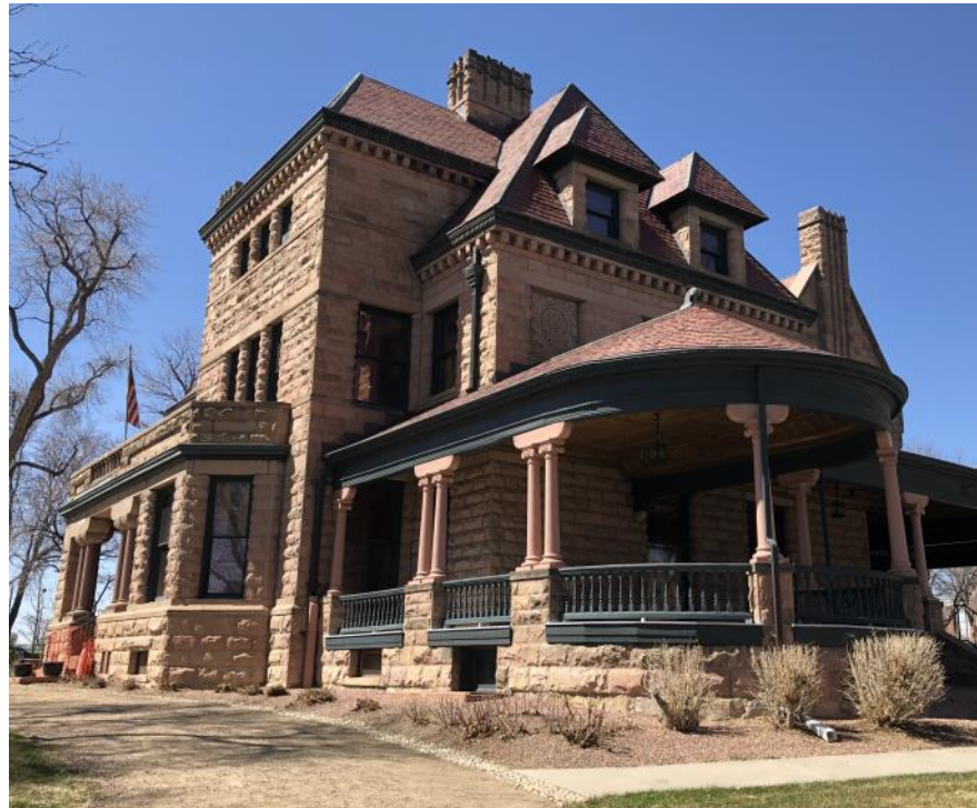
The Rosemount house has 37 rooms over three floors for a total of 24,000 ft 2 !
