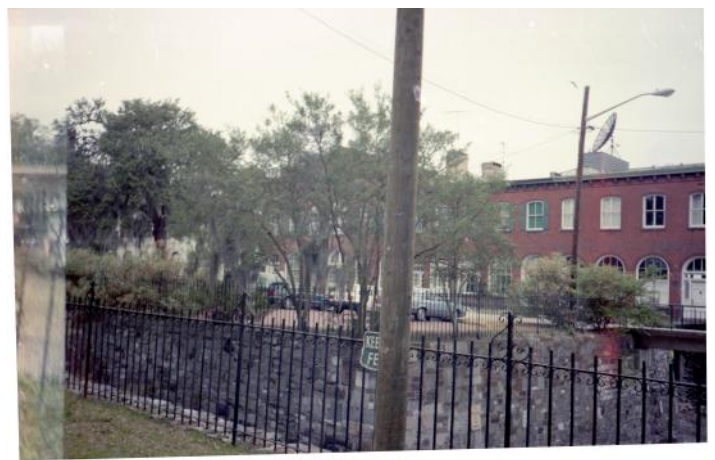
Another view of the Lincoln Street Ramp
