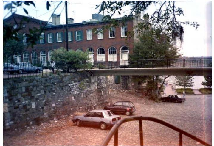
Lincoln Street Ramp.
