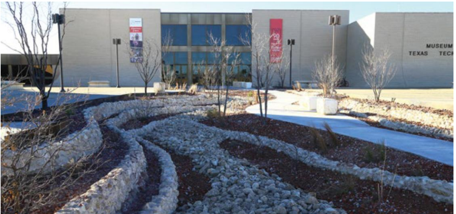
This photo by the Museum shows the arroyo after completion in 2019.
