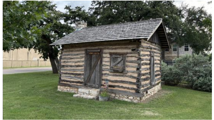
Front view of the cabin, different from the cover photo. This cabin has two doors and two windows.
