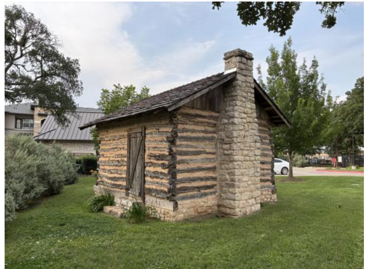
The chimney is local limestone, as is the foundation.
