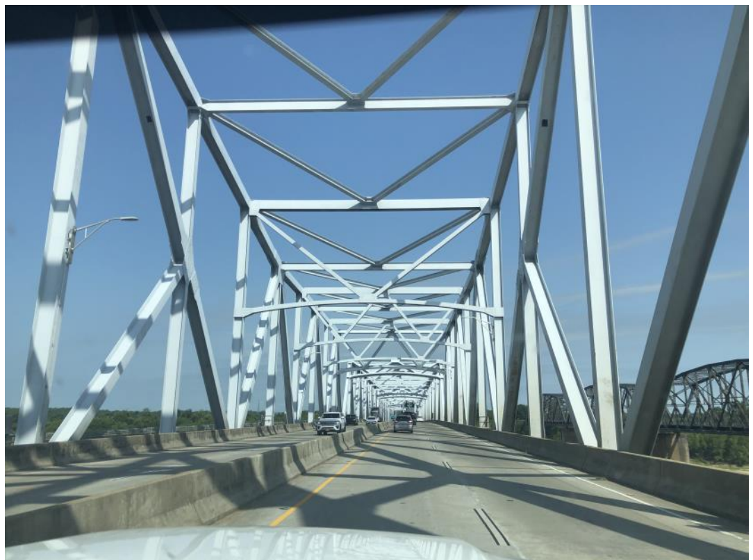
Metal truss bridge over the Mississippi River from Mississippi to Louisiana.
