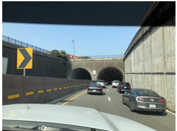
Eastbound entrance of the George Wallace Tunnel.
