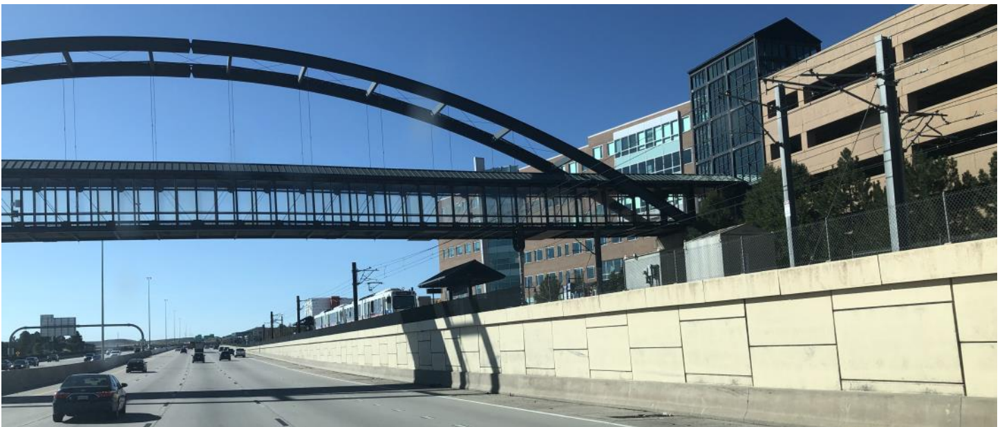
Denver has a light rail commuter train of several routes going all over the Denver metroplex. This is the Lincoln Station in Lone Tree with a cool truss pedestrian bridge.
