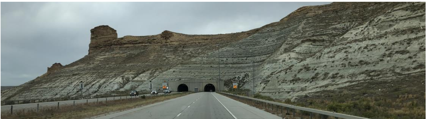
This is the Green River Tunnels located right at the edge of the town of Green River, Wyoming located by the Green River. The tunnel is 1138' through a rock ridge.
