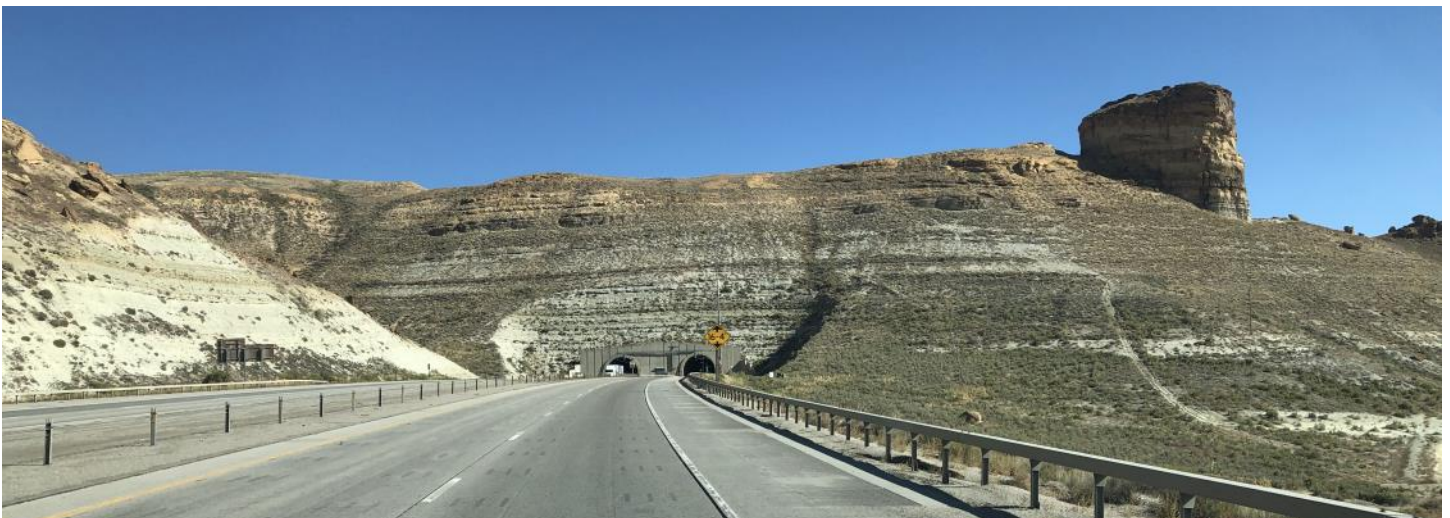
These are the tunnels going through the mountain in Green River, Wyoming.
