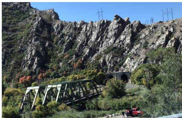
I quickly got this photo of these double train tunnels with truss bridges in an area east of Ogden, Utah.
