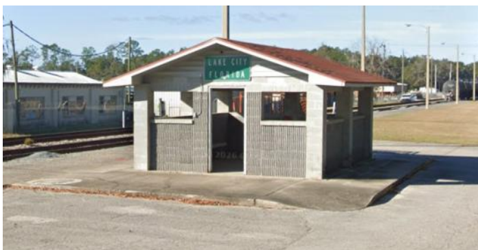
Train station in Lake City, Florida.
