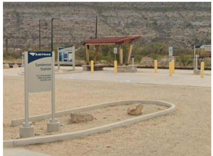
Modern Amtrak stop in Sanderson, Texas. Google Street View
