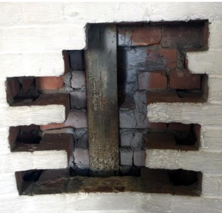
Reinforcing of lighthouse walls
