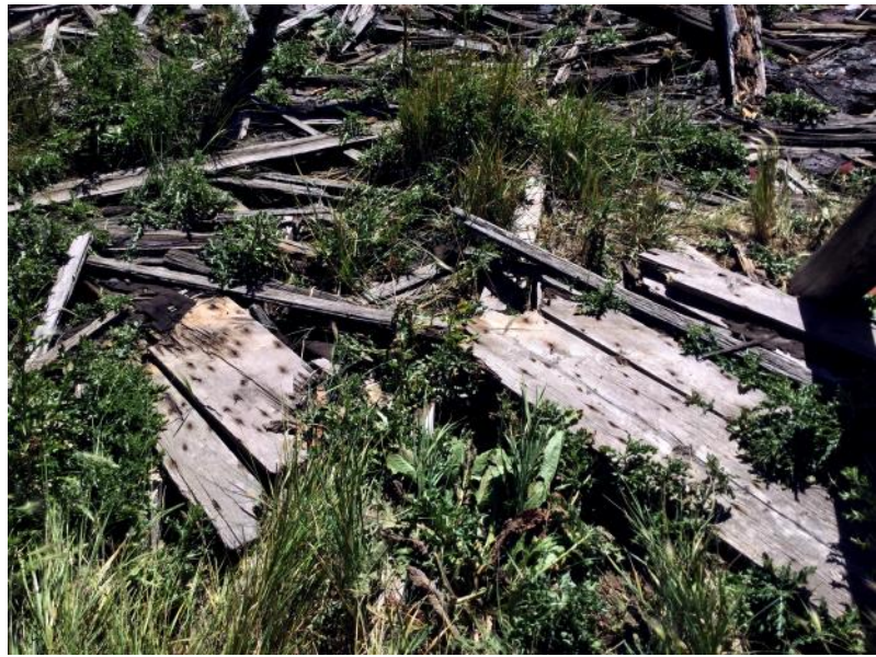
You can see the floor boards running diagonally across the floor joists here near the front door.
