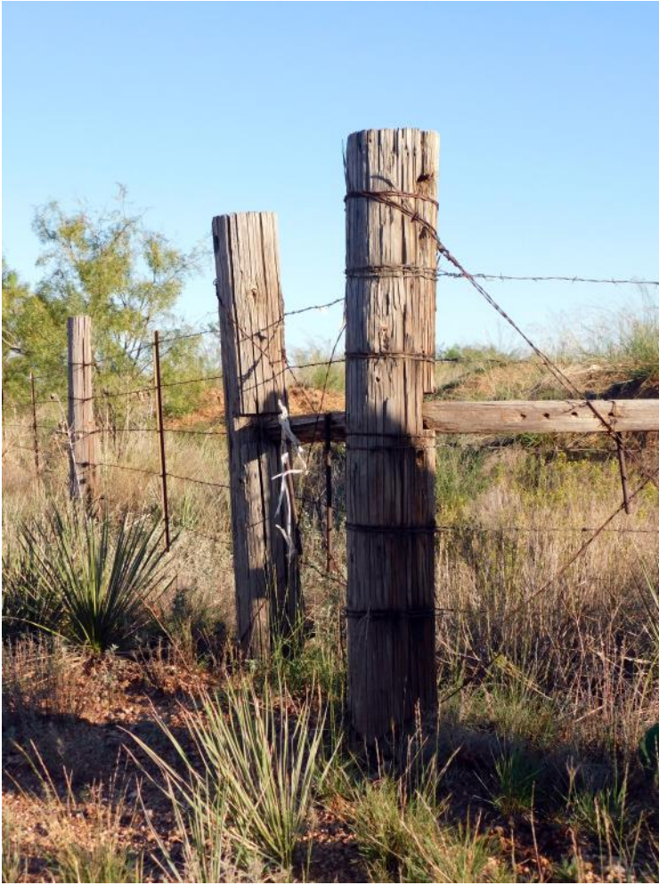
Corner fence post with reinforcing, barbed wire, of course!
