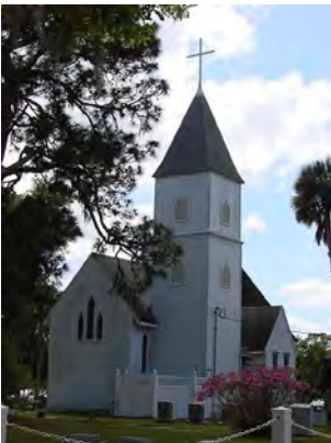
St. Luke's Episcopal Church Courtenay, Florida
