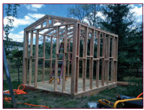
Framing the shed.
