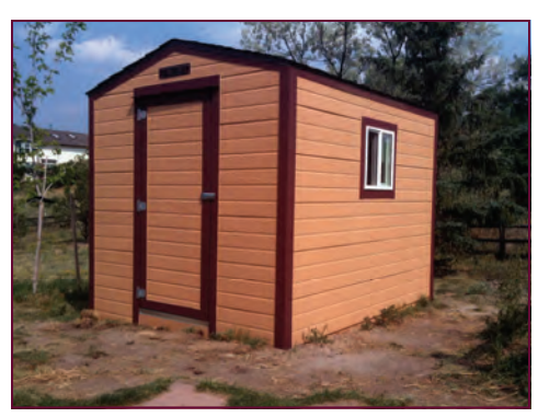
The finished shed.
